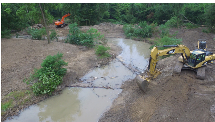
Log structures called cross veins are used to slow and direct water flow
