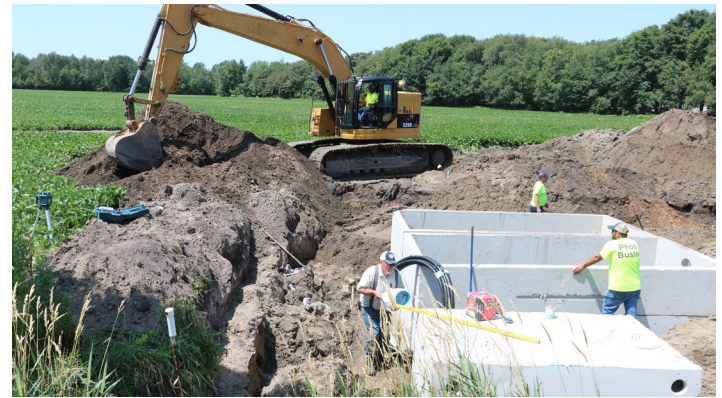
Installation of a large slag filter complex on a field in Fillmore Township
