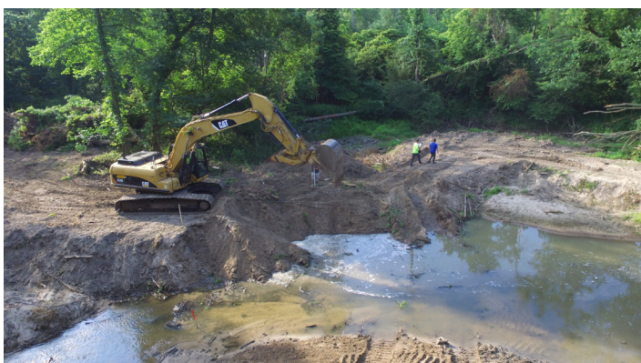
Once banks were cut, logs and brush were installed
