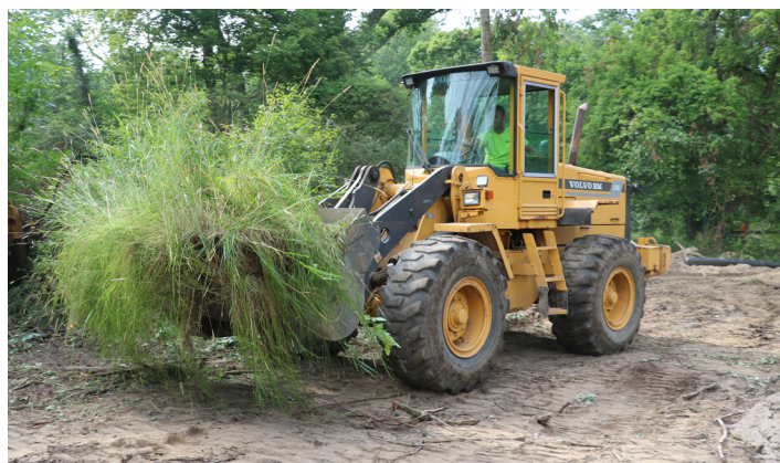
Bringing in mats of grass and shrubs to plant on top of stabilizing banks
