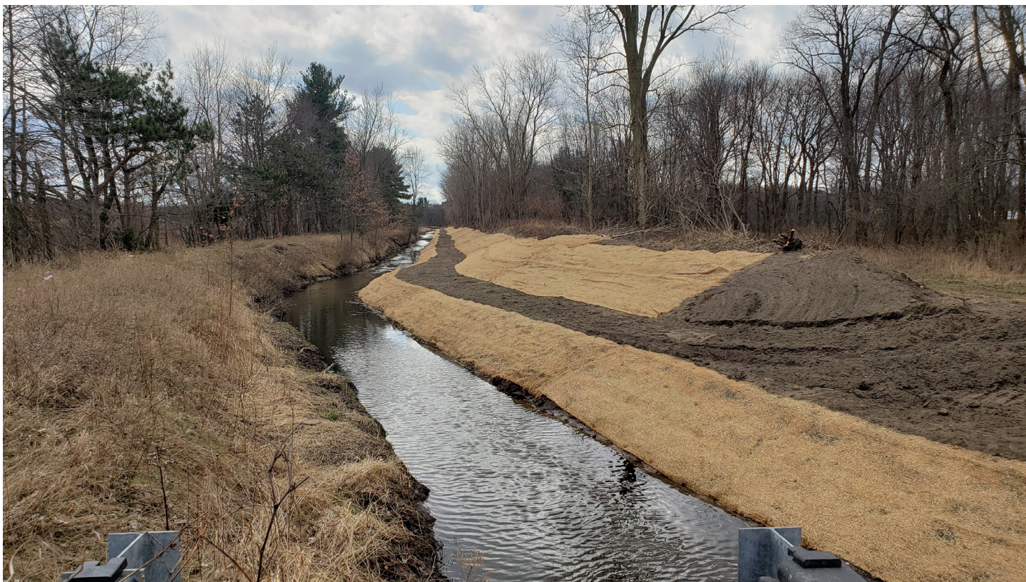
Project Clarity partnered with the Ottawa County Water Resources Commission to construct nearly a mile of two-stage channel on the Harlem Drain in Park Township. Matching funds from the township made this project possible.
