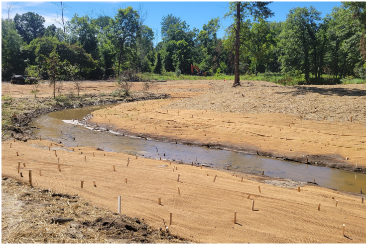
July - erosion blankets staked
