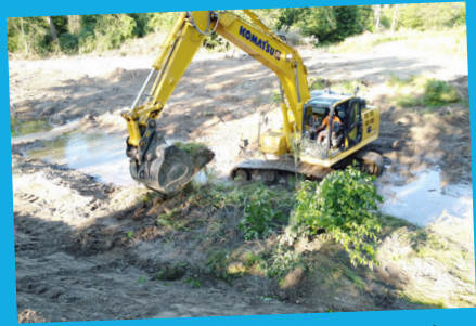
Reshaping stream banks in preparation for erosion mats and native planting.
