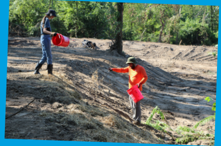
Spreading native straw and seed along the bank.
