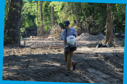
Spreading native straw and seed along the bank.
