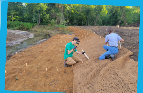
Placing stakes that keep erosion mats in place.
