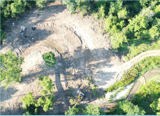
Reshaping stream banks in preparation for erosion mats and native planting.
