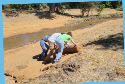
Rolling out biodegradable mats that hold seeds and straw in place until they become better established.
